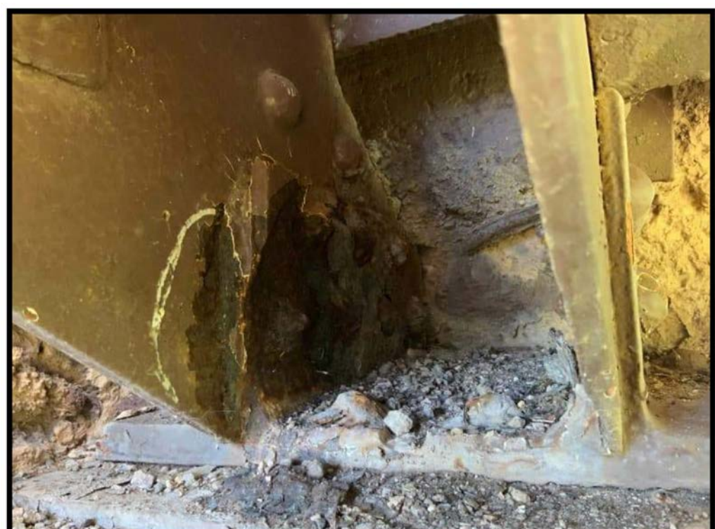
Corrosion and severe section loss at bridge bearing pockets
